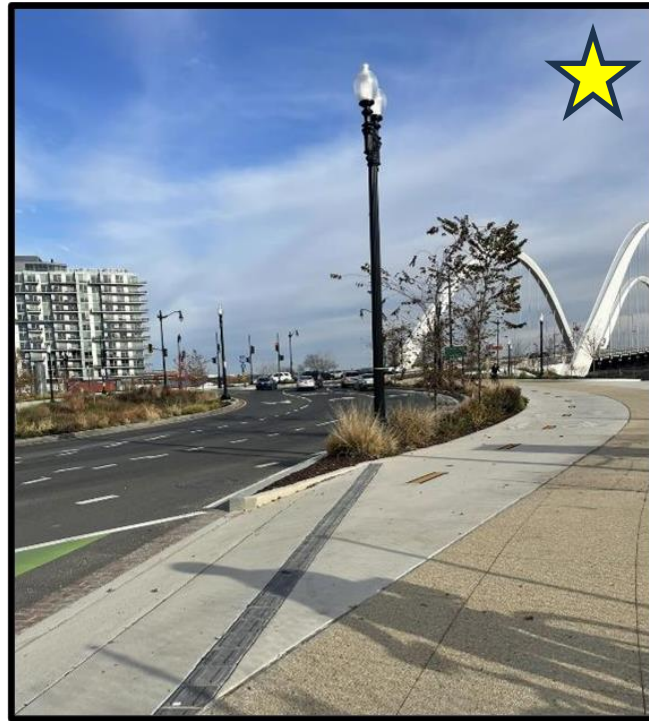
Existing facility at Frederick Douglass Memorial Bridge
